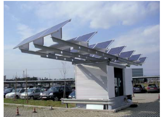
Vanadium redox battery with photovoltaic panels as RAPS
