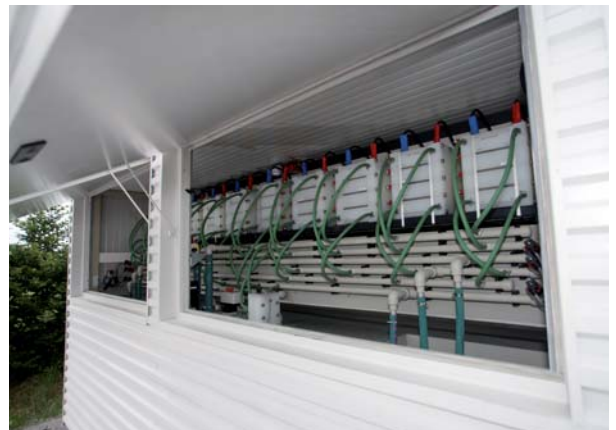
View of the reactors of the system FB10/100
