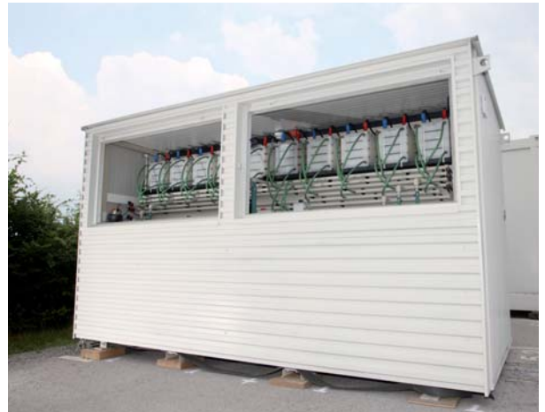
General view of the system FB10/100
